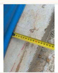
Steel frame bottom plates are overhung more than the maximum allowance of 10mm in one or more areas of the slab. Non-shrinkage cement-based material to be applied to the side of the slab rebate to cover under the bottom plate.
