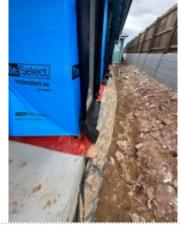
Some parts of physical termite barrier damaged or installed improperly. Fixing required.
